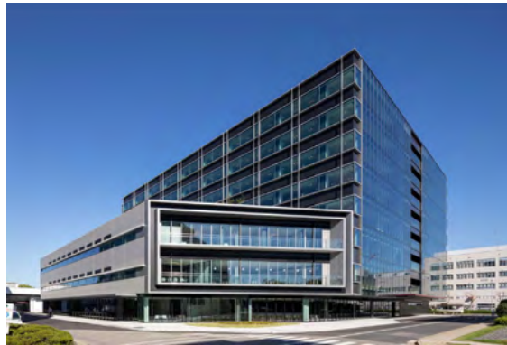
Research and Development Building
