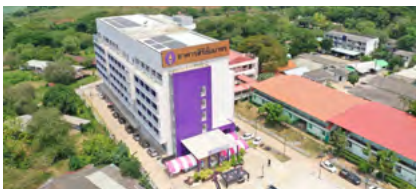
Hospital with a rooftop solar power system installed as part of the "Solar for Lives" environmental project
