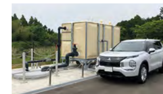
Power being supplied on a trial basis by a plug-in hybrid electric vehicle
