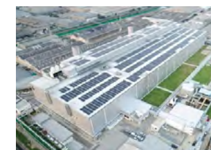
New paint plant (MTh)
