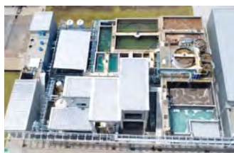
Wastewater recycling plant (MMTh)
